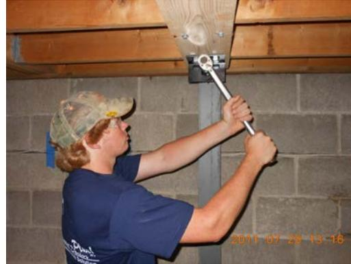
**11)** Place the top bracket with compressed spring against the face of the beam and mark the two holes in the bracket. Remove the bracket and drill out the holes through the 2" x 8". Try to keep the holes near the center of the 2" x 8". Bolt the top bracket in place. Now follow steps 7 and 8.
