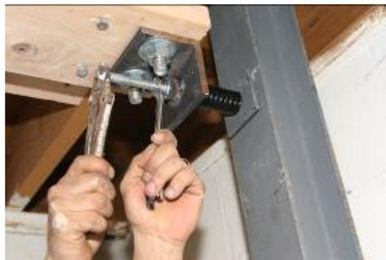
8) Install the 3/4" seating bolt and tighten it using a torque wrench set at 40 pounds. Again start at the middle and work to the ends. **If the spring does not align directly with the bolt**, use a small punch or screw driver and hammer to re-position the bearing plate to allow the seating bolt to cleanly pass through the spring.
