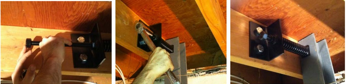
9) **Floor joist running parallel to the wall:** Completing steps 1 through 5. Solid blocking is required. The blocking should consist of the same dimension lumber that the floor joists are made of and should extend back a minimum of three joists from the wall. Use nails and screws to secure the wood in place.
