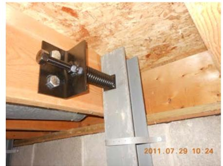
7) Carefully remove the compression bolt by holding the all-thread with a pair of vise grips and turning the nut. This will prevent the all-thread from backing out of the assembly nut. The tension can be slowly applied to the beam by loosening the nut. Start in the middle of the wall and work to the ends rotating back and forth from one beam to the other. Once the nut has been completely loosened, remove the all-thread from the bracket.
