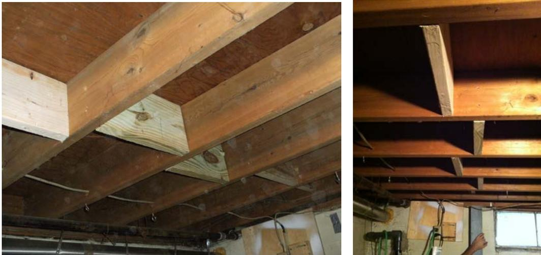
**10)** Once the solid blocking is in place, attach a 2"x 8"x 8' long board to the bottom of the floor joists. Bolt the 2' x 8' to the bottom of the floor joist using two 3" long by 3/8" diameter zinc-coated lag screws with washers in each floor joist. You should first tack the 2x8 to the floor joist using nails so you can drill pilot holes in the joists to prevent splitting.
